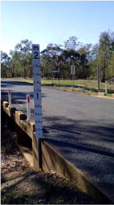
Image 87: Flood Depth Indicator west of Structure 31.
