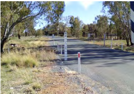
Image 88: Flood Depth Indicator east of Structure 28.
