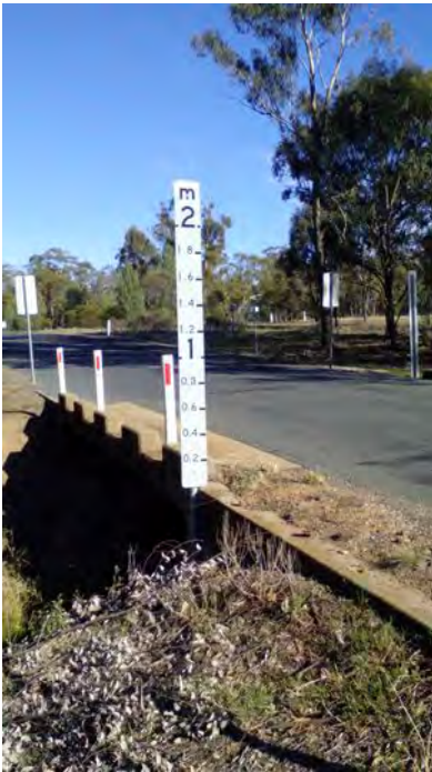
Image 86: Flood Depth Indicator East of Structure 31.
