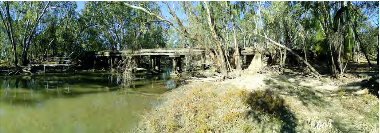
Image 41: Structure 16 facing downstream.
