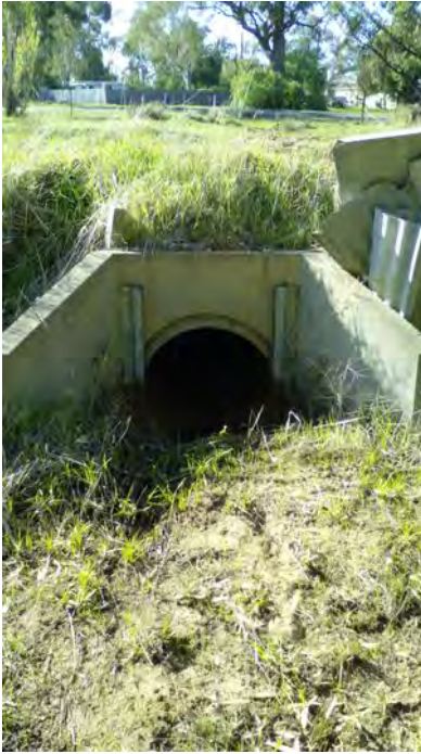
Image 123: Rand Levee Bank, 600mm rcp outlet.
