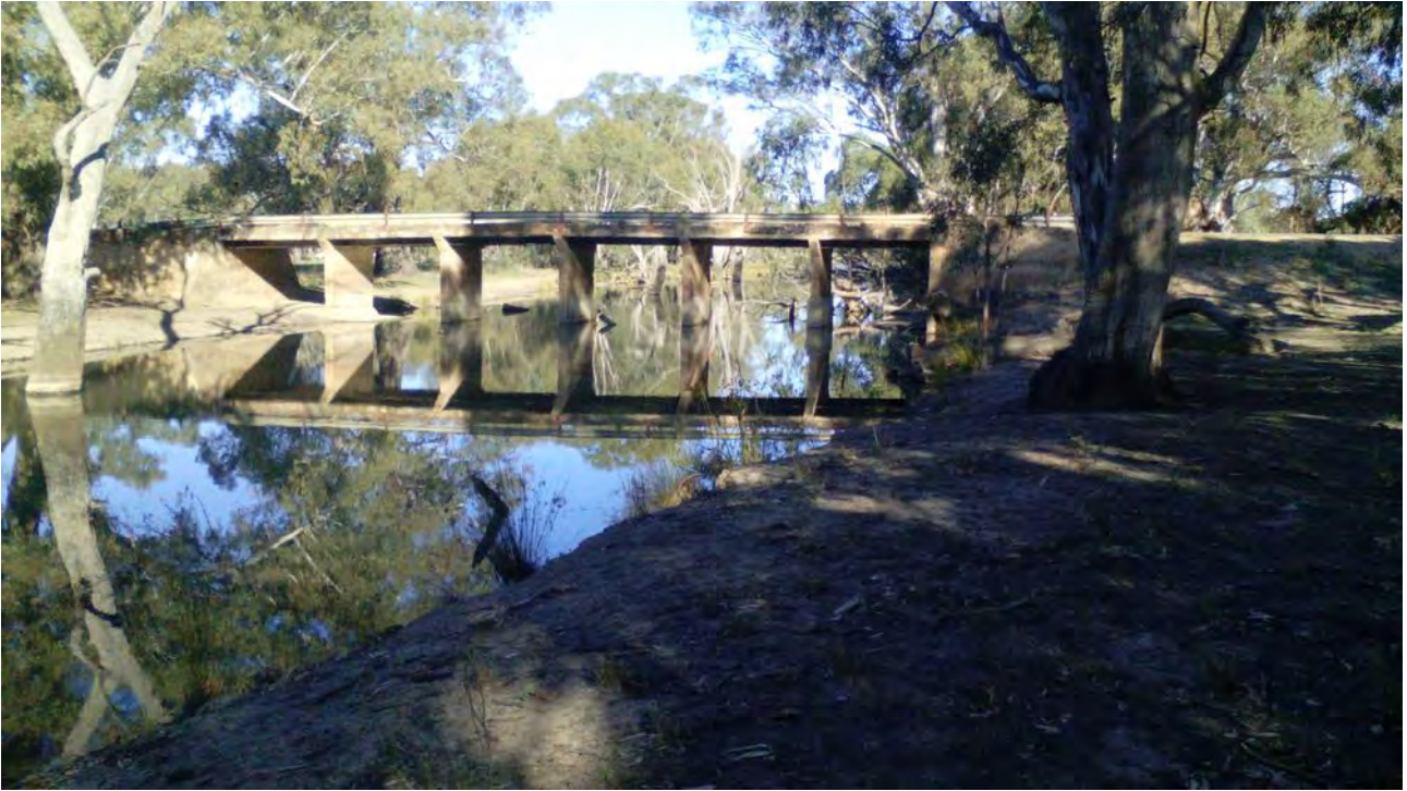
Image 51: Structure 21 facing downstream.
