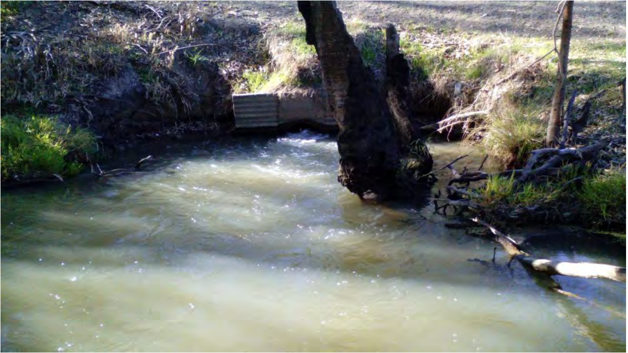
Image 36: Structure 13 facing upstream.
