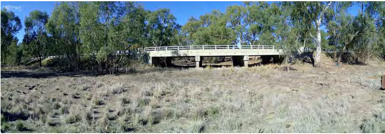
Image 47: Structure 19 facing downstream.
