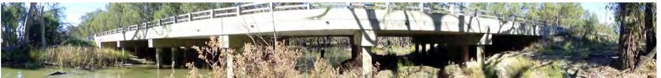
Image 43: Structure 17 facing downstream.
