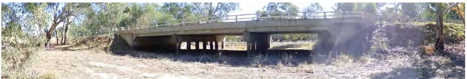
Image 48: Structure 19 facing upstream.
