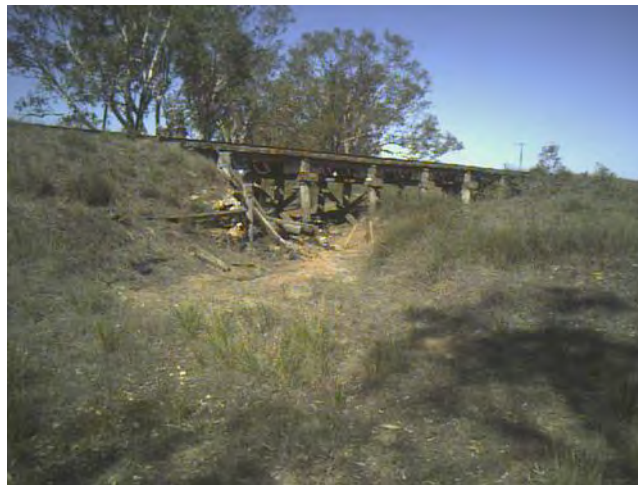
Image 30: Structure 10 facing upstream.
