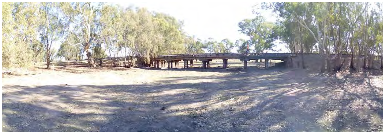
Image 46: Structure 18 facing upstream.
