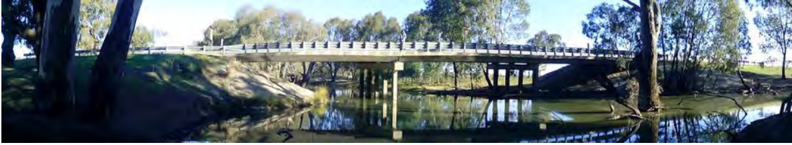
Image 49: Structure 20 facing downstream.
