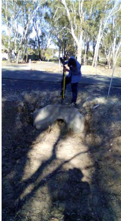
Image 39: Structure 15 facing downstream.
