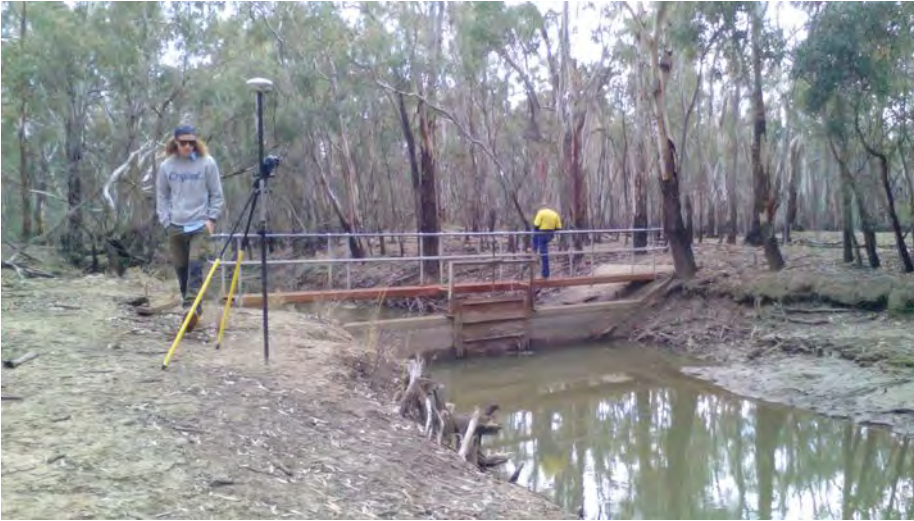
Image 132: Spiller's Regulator facing downstream.
