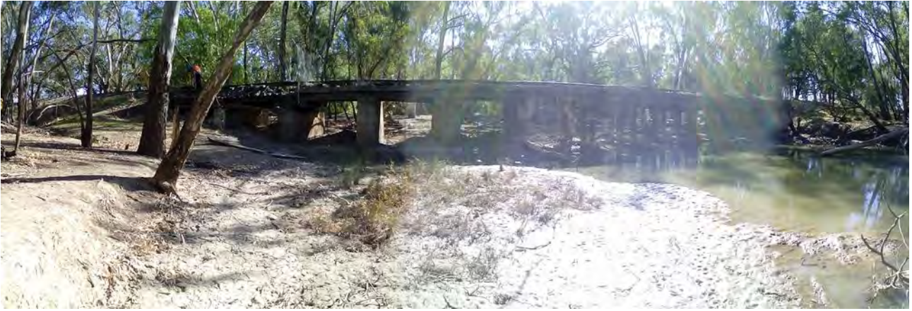
Image 42: Structure 16 facing upstream.
