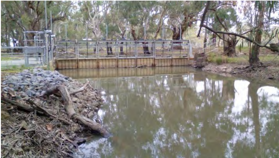
Image 124: Tarabah Weir facing downstream.
