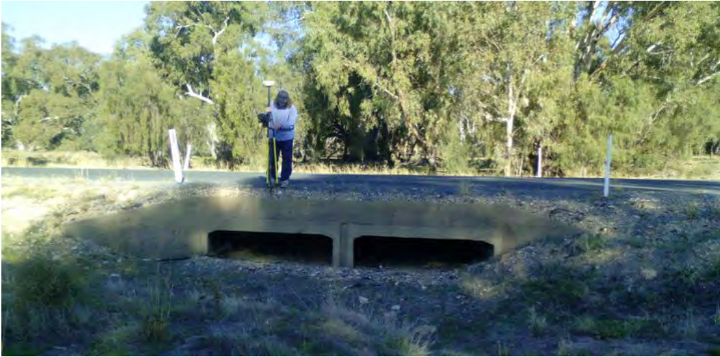
Image 33: Structure 12 facing downstream.
