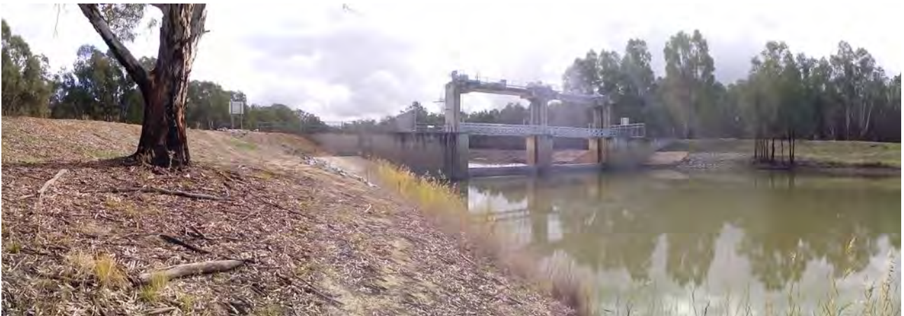
Image 128: Yanco Weir facing downstream.
