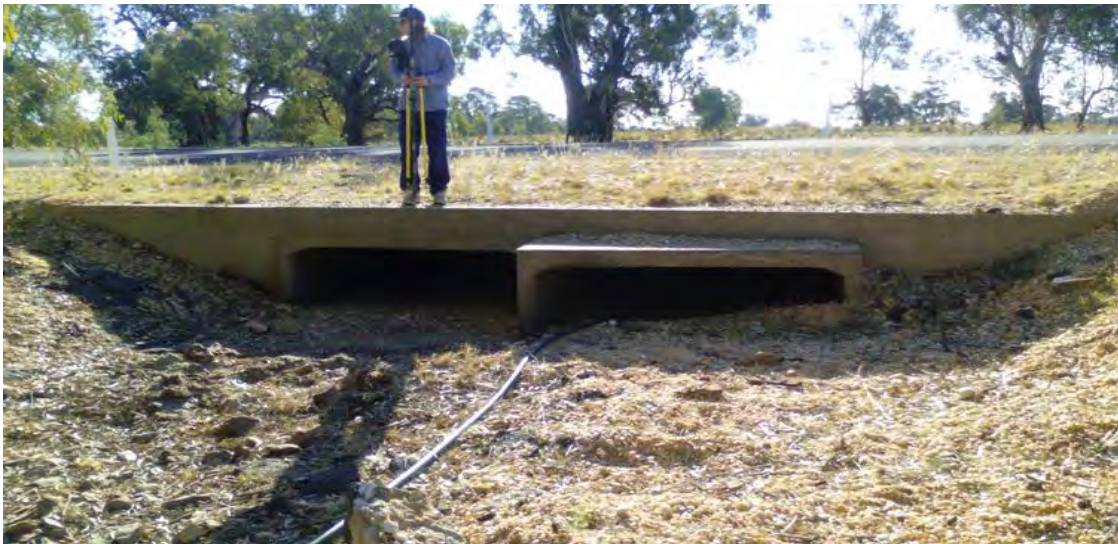
Image 34: Structure 12 facing upstream.
