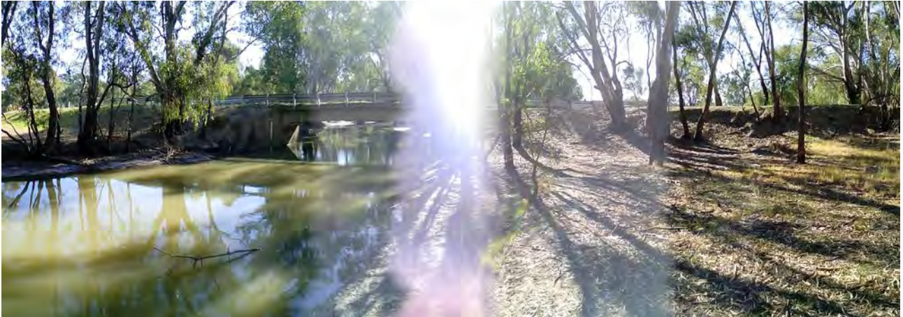
Image 38: Structure 14 facing upstream.
