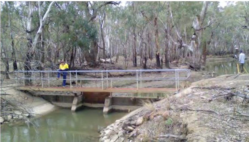
Image 133: Spiller's Regulator facing upstream.
