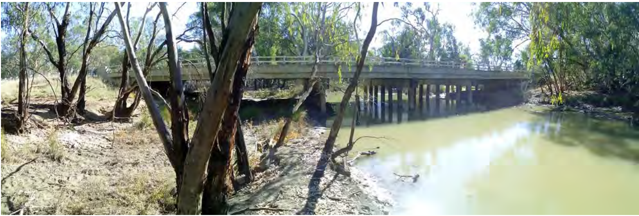
Image 44: Structure 17 facing upstream.
