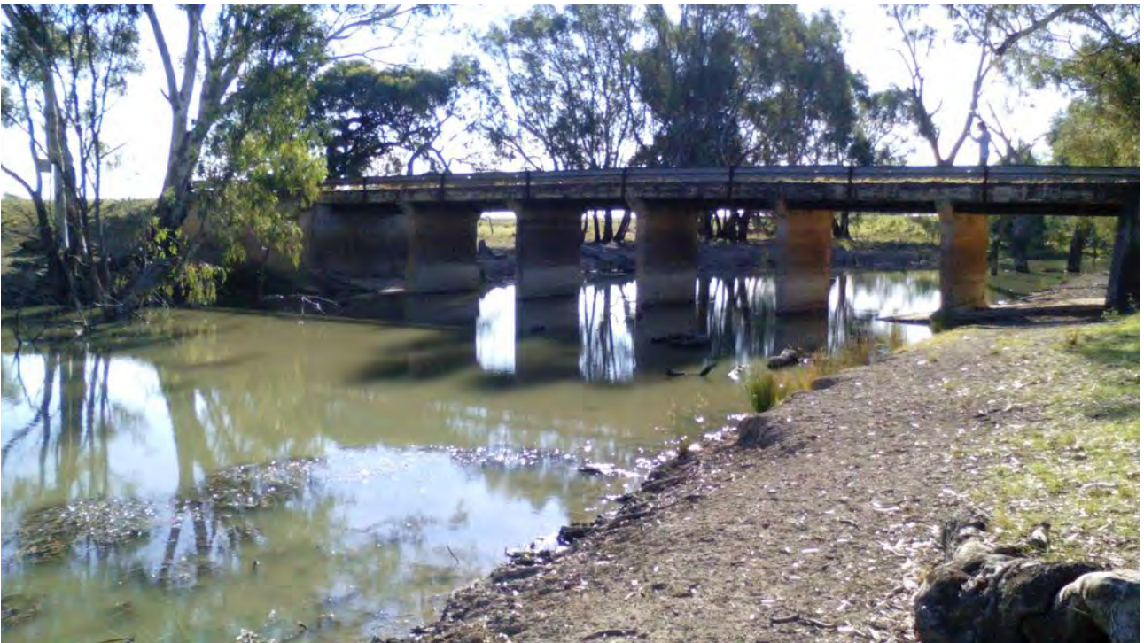
Image 52: Structure 21 facing upstream.
