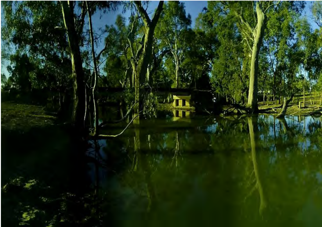
Image 32: Structure 11 facing upstream.
