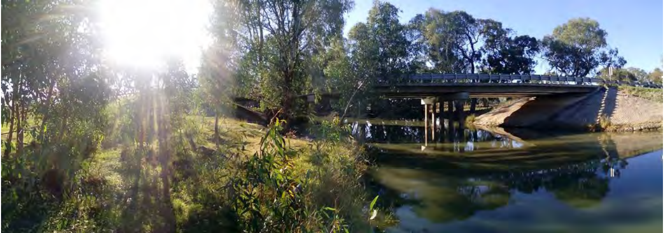
Image 50: Structure 20 facing upstream.
