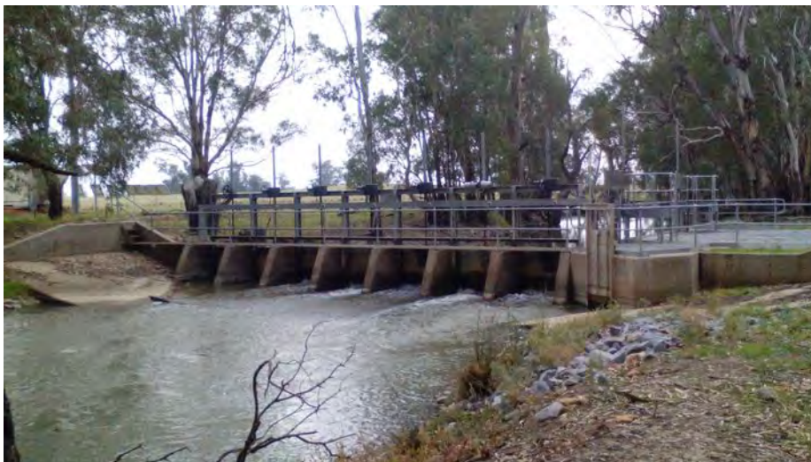
Image 125: Tarabah Weir facing upstream.
