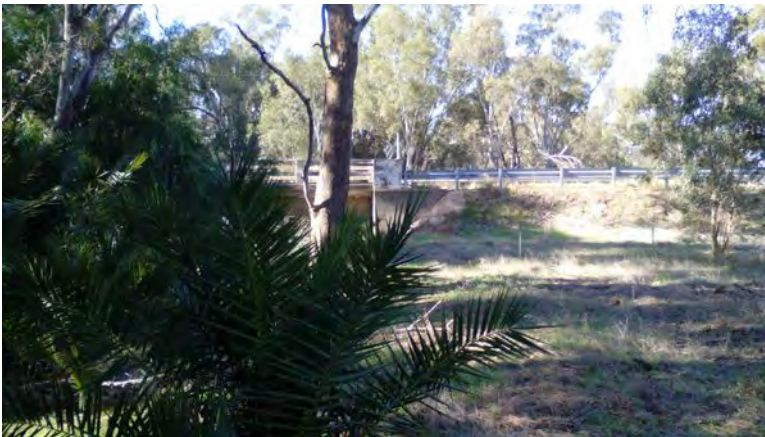
Image 80: Structure 35 facing upstream.
