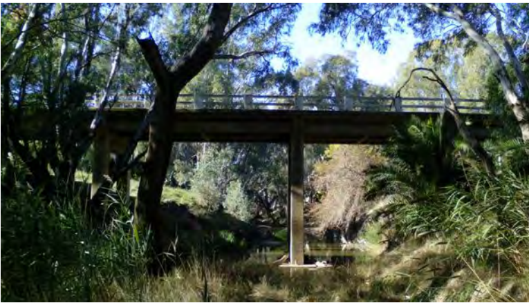
Image 80 shows structure 35 facing upstream.
