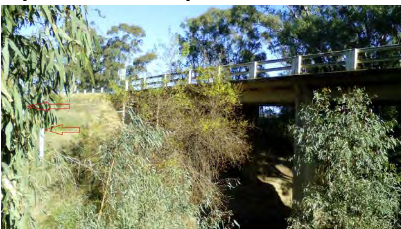
Image 85: Flood depth Indicators near bridge 35, Rand.
