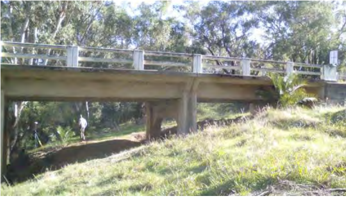
Image 79: Structure 35 facing downstream.
