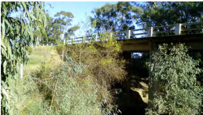
Image 77: Structure 35 facing downstream.
