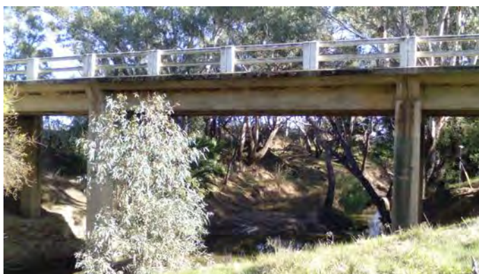
Image 78: Structure 35 facing downstream.
