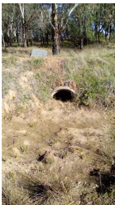
Image 122: Rand Levee Bank, 600mm rcp inlet.
