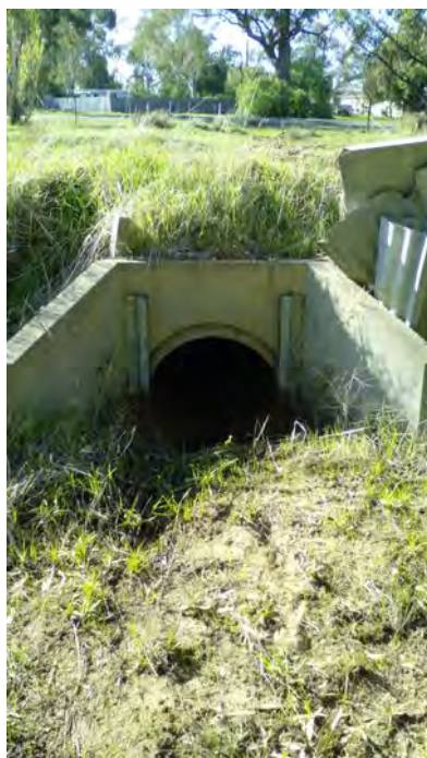
Image 123: Rand Levee Bank, 600mm rcp outlet.
