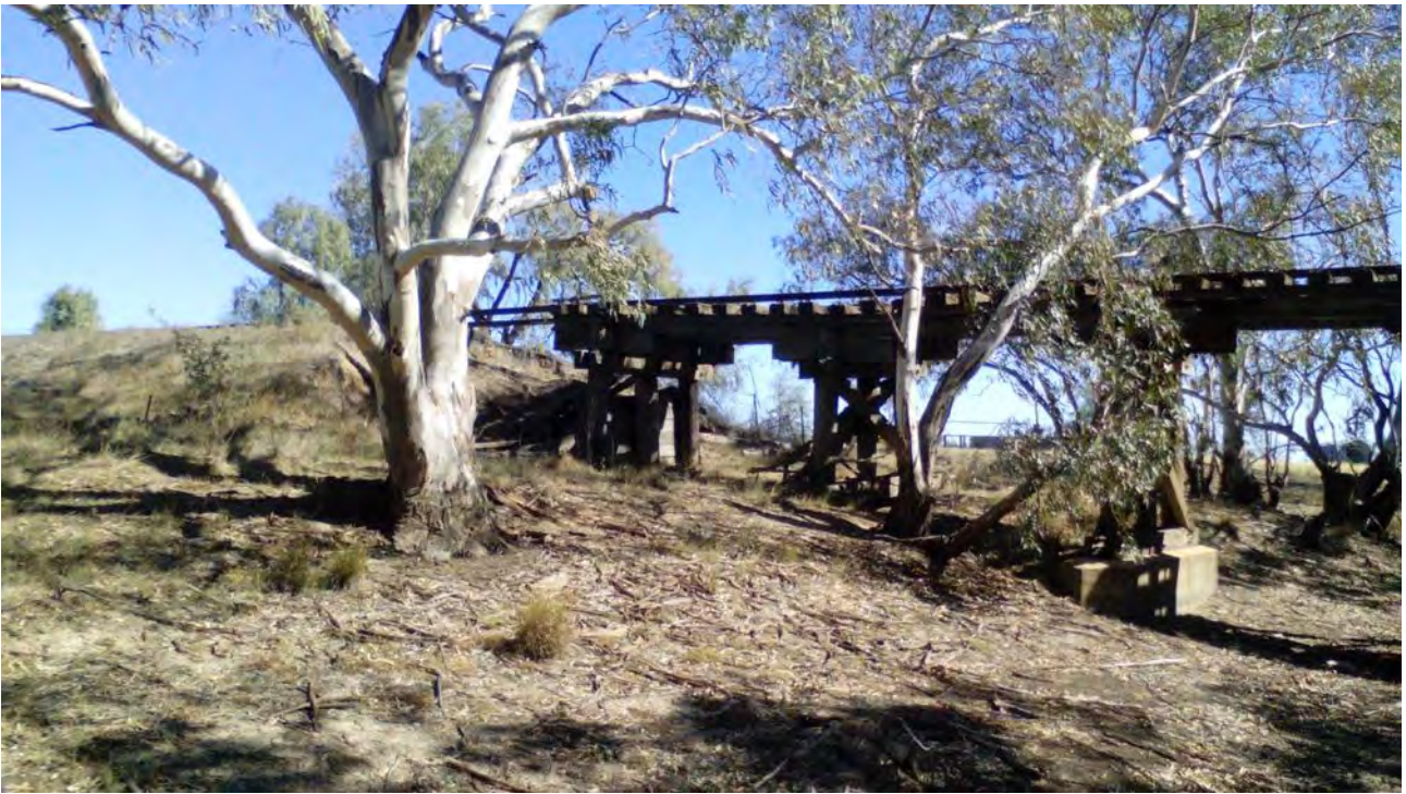
Image 24: Structure 9 facing downstream.
