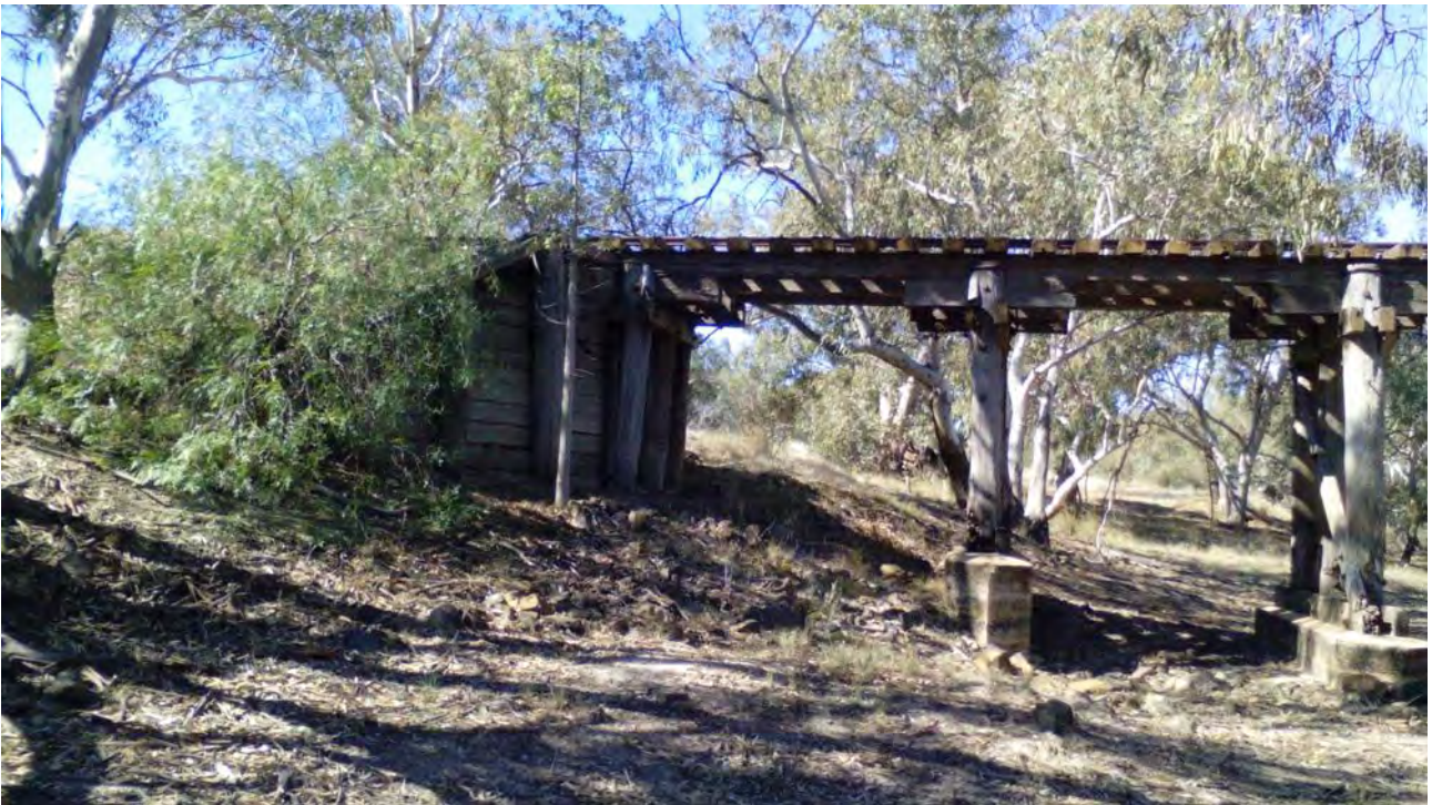
Image 25: Structure 9 facing upstream.
