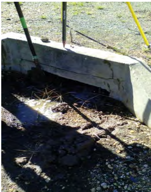
Image 10: Structure 4 facing downstream.
