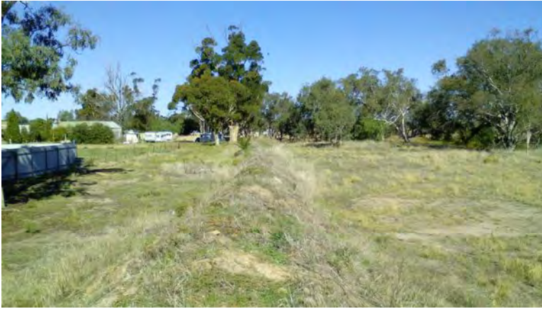
Image 97: Urana Levee Bank.
