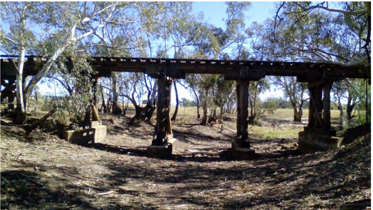
Image 23: Structure 9 facing downstream.
