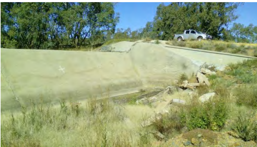
Image 96: Urana Dam Spillway.
