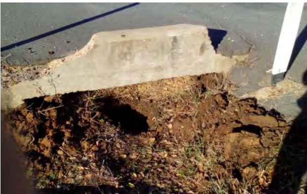
Image 107: North-West Intersection of Chapman and William Street facing East. This culvert seems to be on strip footings with earth as its base.
