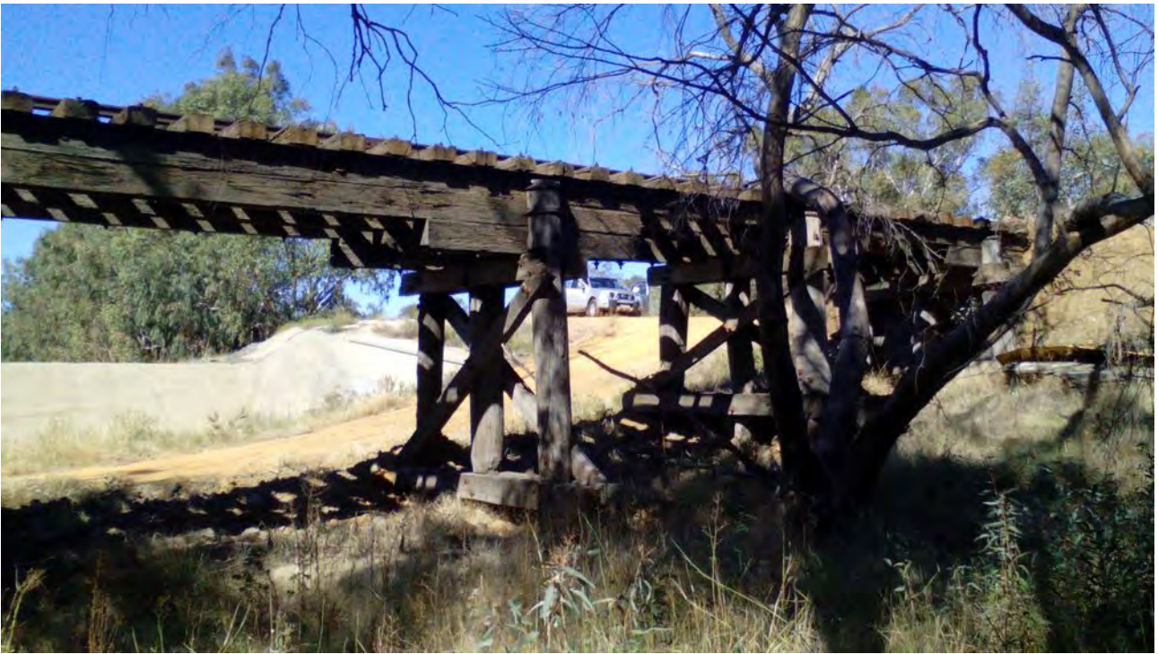
Image 21: Structure 8 facing upstream.
