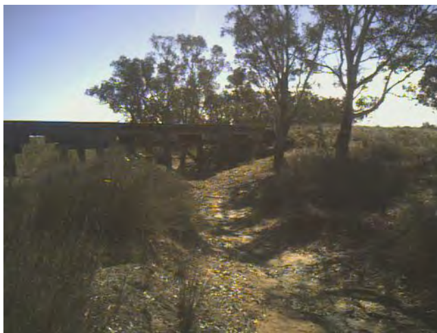
Image 28: Structure 10 facing downstream.
