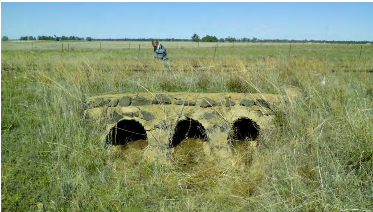
Image 15: Structure 7 facing upstream.
