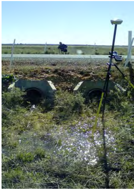
Image 13: Structure 6 facing downstream.
