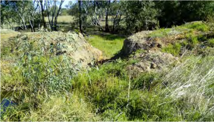
Image 100: Urana Levee Bank washout at Osborne Street.
