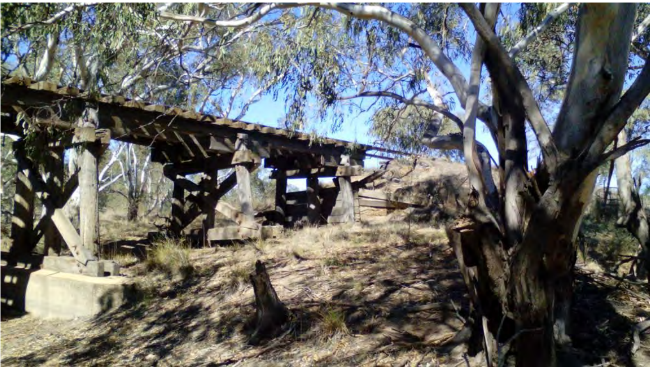
Image 27: Structure 9 facing upstream.
