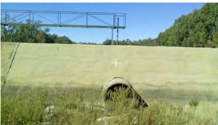
Image 94: Urana Dam Spillway outlet.
