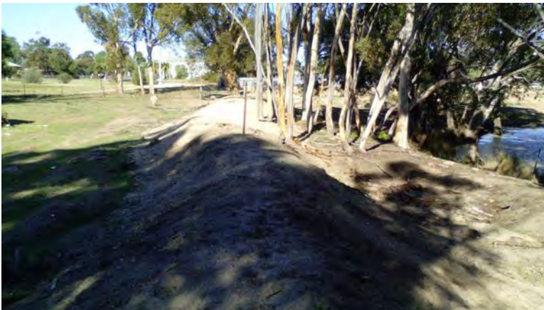
Image 98: Urana Levee Bank.
