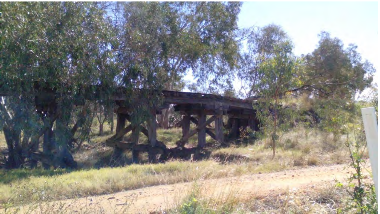
Image 18: Structure 8 facing downstream.
