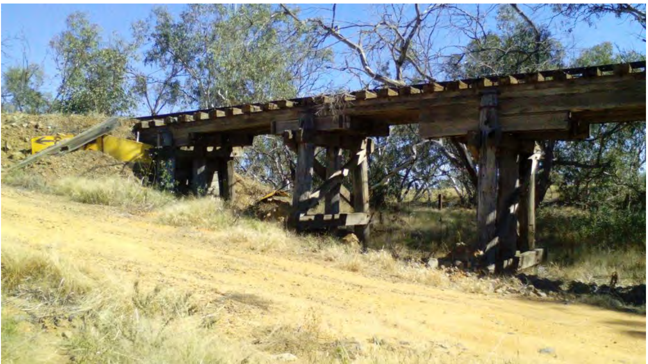
Image 16: Structure 8 facing downstream.
