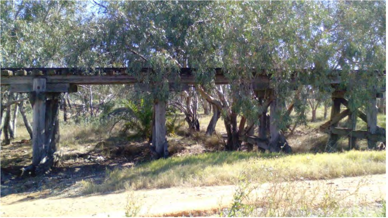
Image 17: Structure 8 facing downstream.
