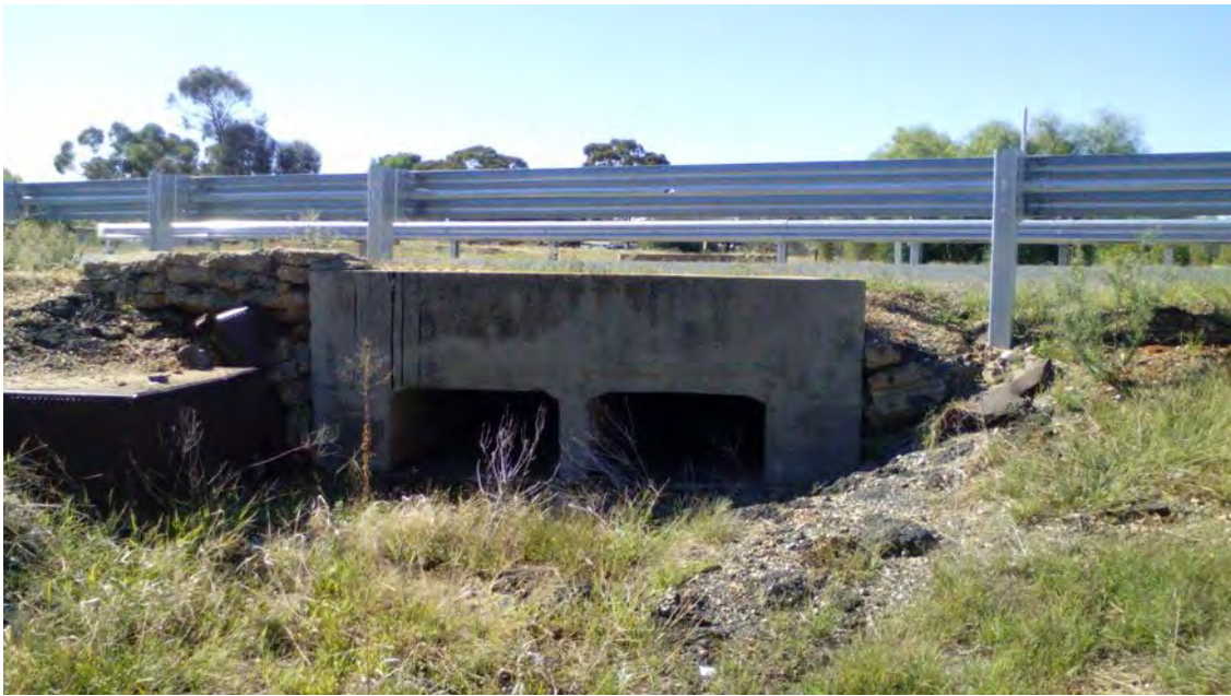
Image 12: Structure 5 facing upstream.
