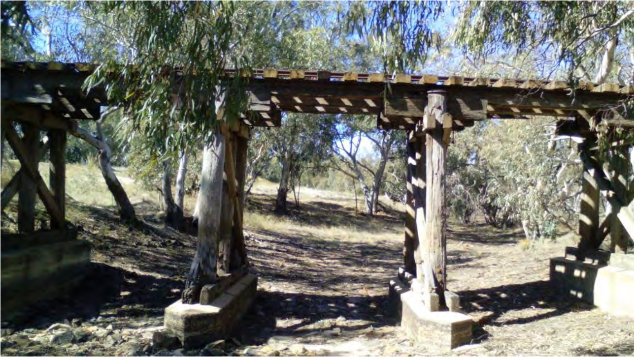
Image 26: Structure 9 facing upstream.
