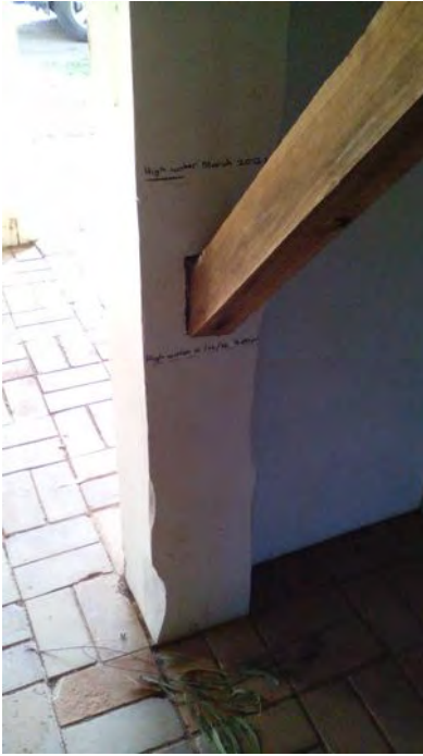
Image 90: Flood Marks at Emro.
