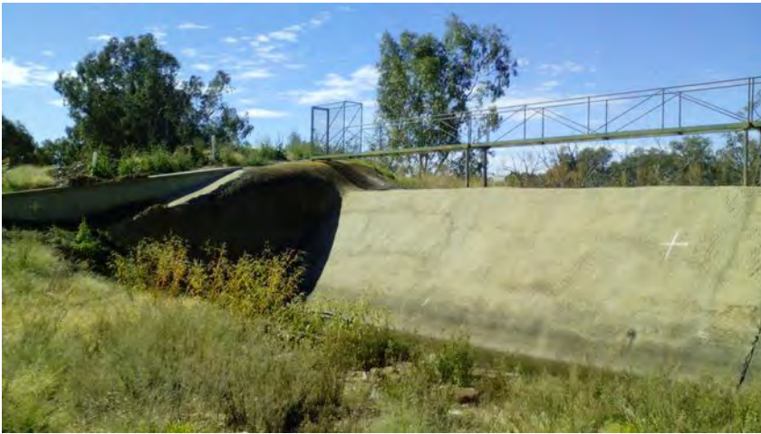
Image 95: Urana Dam Spillway.
