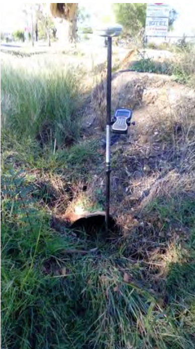
Image 109: Outflow of Chapman Street Storm-water system.
