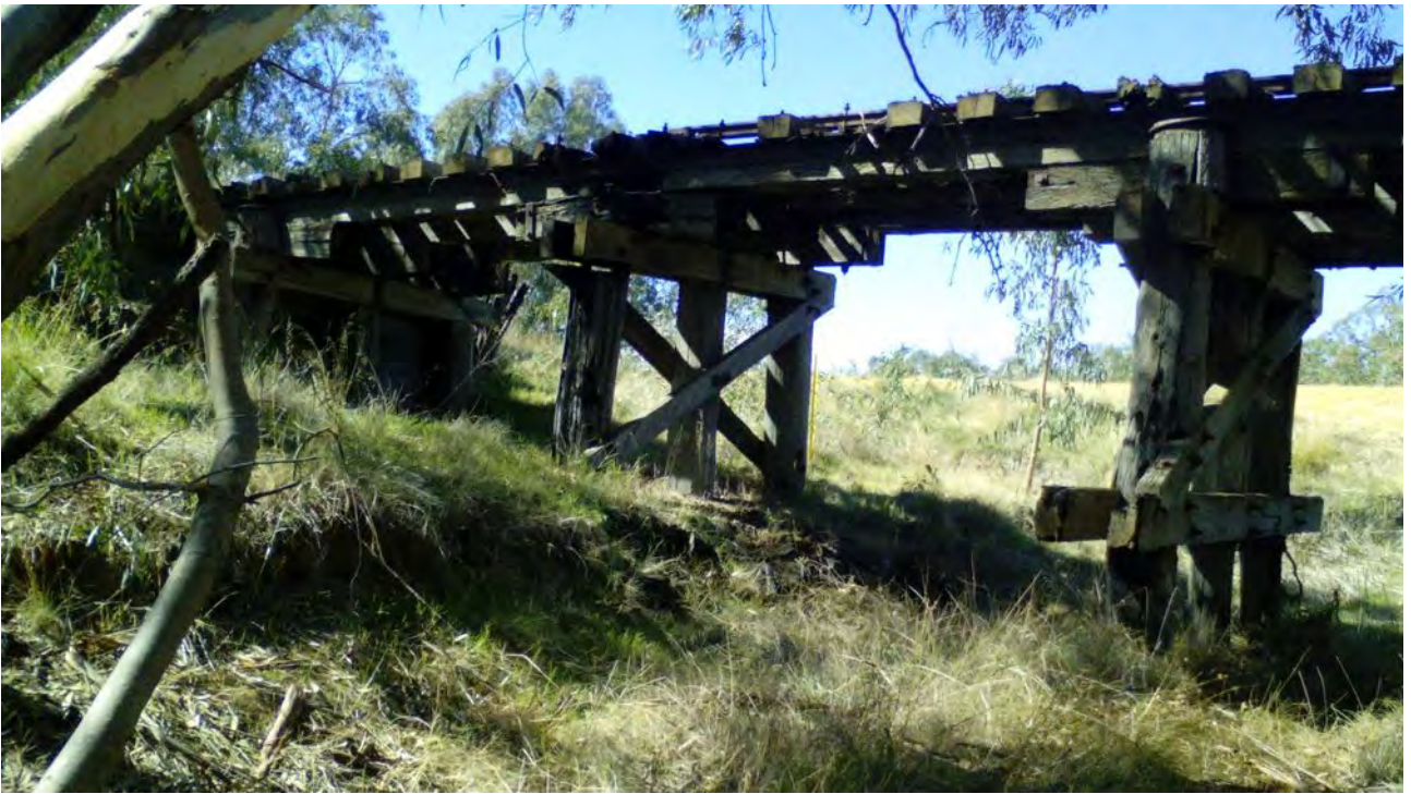
Image 19: Structure 8 facing upstream.
