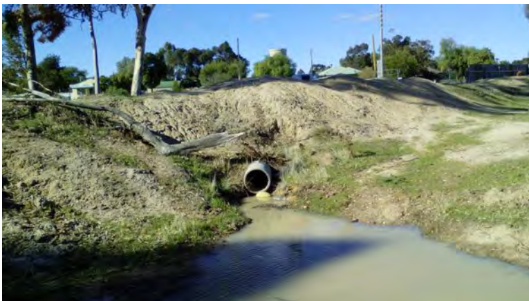
Image 102: Outlet of 375mm RCP at the continuation of Stephen Street.
