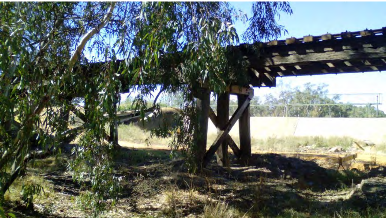
Image 20: Structure 8 facing upstream.
