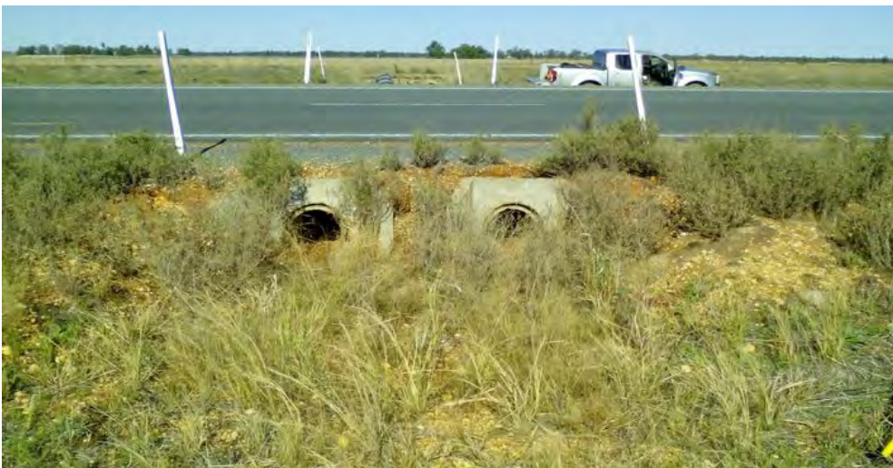
Image 14: Structure 6 facing upstream.
