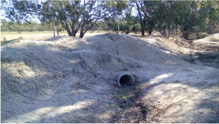
Image 103: Inlet of 375mm RCP at the continuation of Stephen Street.
