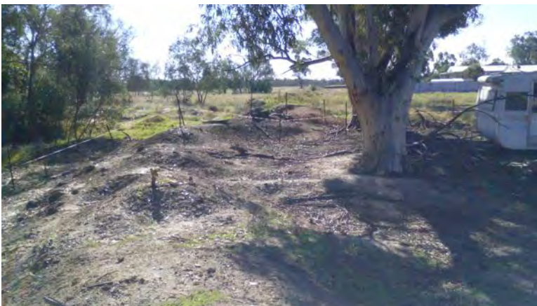
Image 99: Urana Levee Bank so areas are in a state of disrepair.
