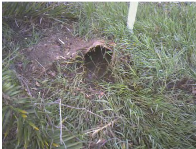
Image 9: Structure 3 facing upstream.
