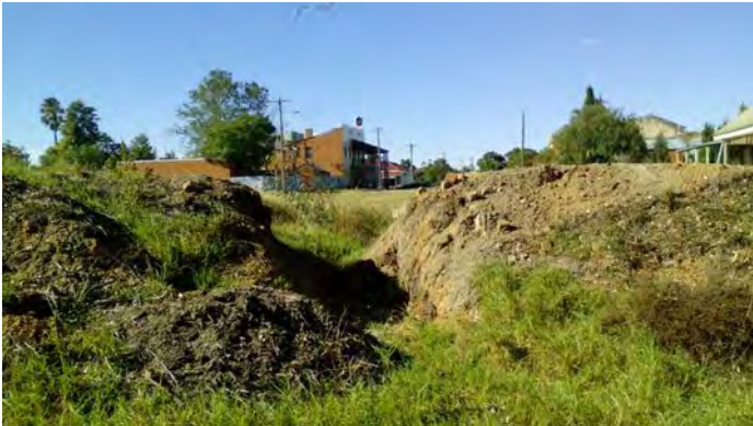
Image 101: Urana Levee Bank washout at Osborne Street.
