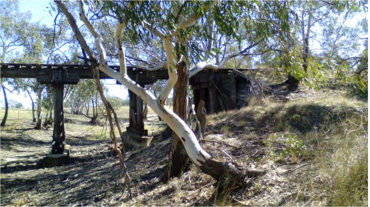
Image 22: Structure 9 facing downstream.
