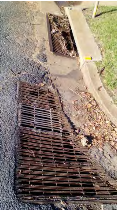
Image 110: Grated storm-water pits at the South-East corner of the Intersection of William and Osborne Streets facing East.
