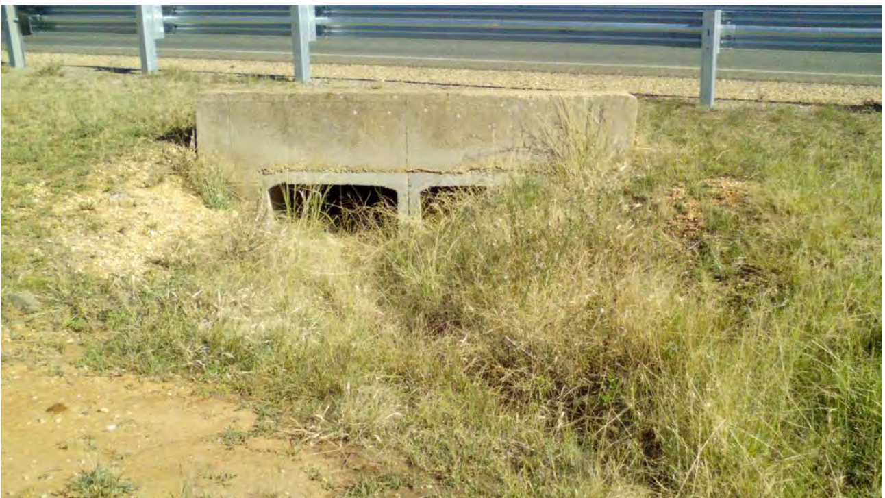
Image 11: Structure 5 facing downstream.
