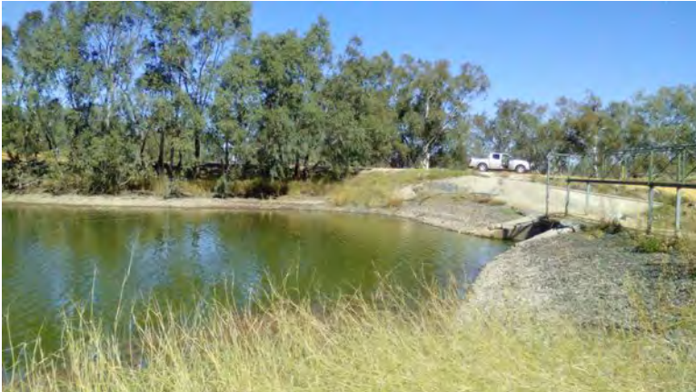
Image 92: Urana Dam Spillway.
