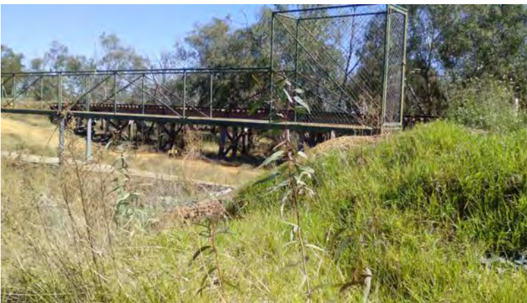
Image 93: Urana Dam Spillway overflow access.
