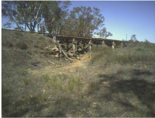
Image 30: Structure 10 facing upstream.
