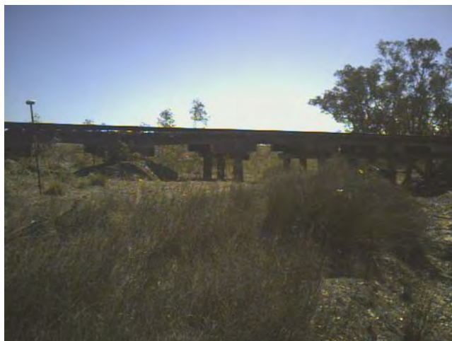
Image 29: Structure 10 facing downstream.
