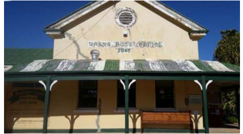
Pictured above: the post office before repainting.
