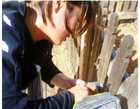
Above: Mimi fixing pickets to the fence
