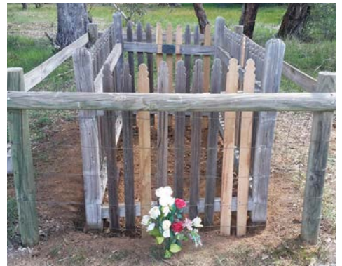
Above: Completed restoration
