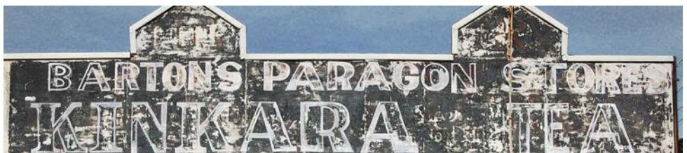
Pictured above: Work began on traces of the parapet signs. Lettering can be set out more accurately when other similar historic signs have been researched.
