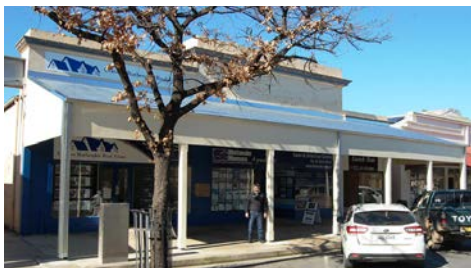
Pictured above: Reframed in timber, the restored verandah utilises recycled timber posts.
