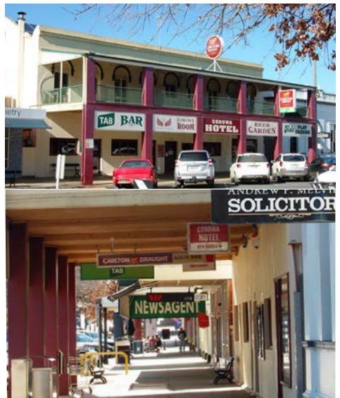
Pictured above: Corowa Hotel's upper floor verandah roof, reframed in timber, stabilised and repainted, makes a big contribution to Corowa's heritage streetscape.
