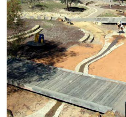
Low bridge over paved swale
