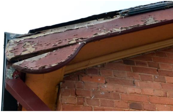
Urana Courthouse – finish painting exterior
