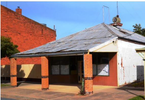
Old café – repair and paint frontage
