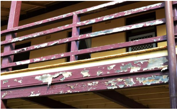
Urana Hotel – paint verandah timbers
