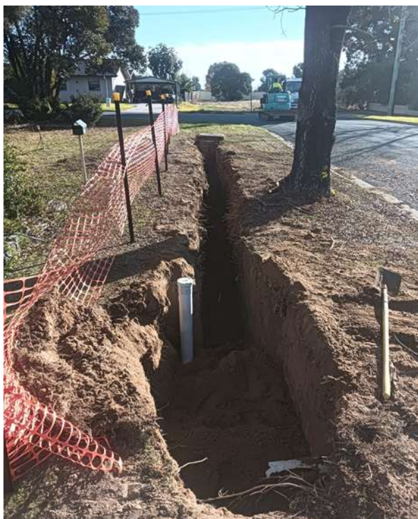
McDonald Avenue Sewer Repair
