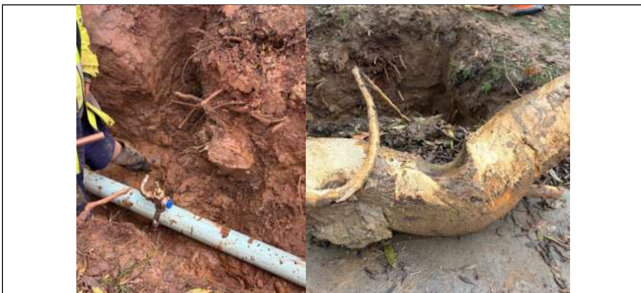
Edwards St, Corowa - Water mains break caused by tree root wrapping around pipe
