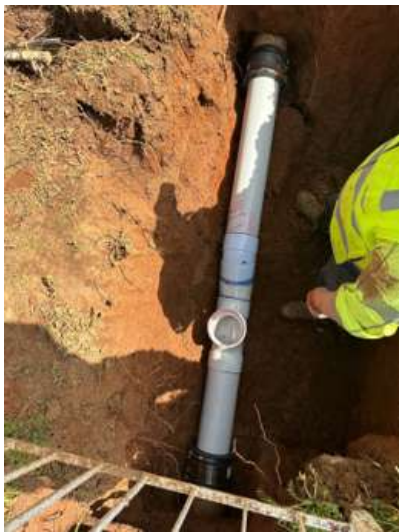
Sewer service rebuild
