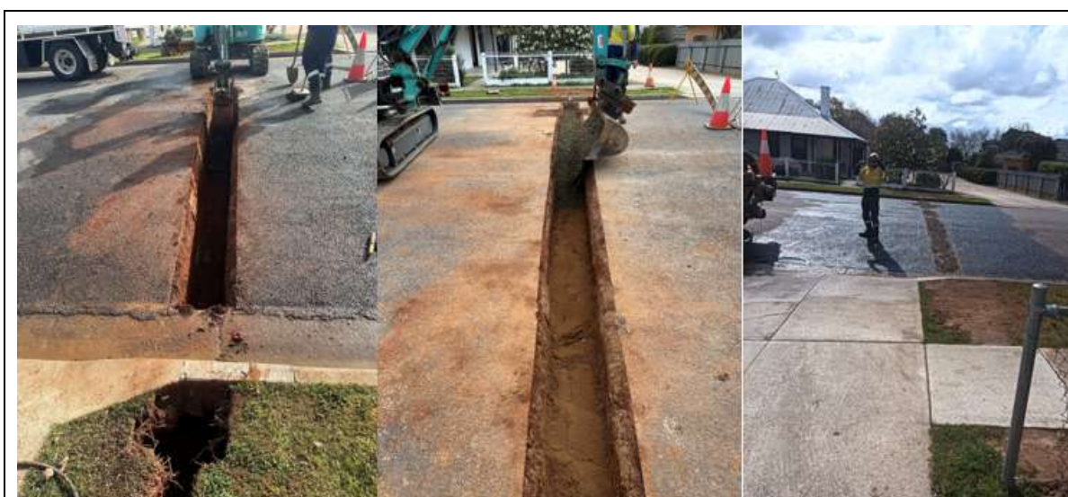
Guy Street Corowa new water connection – (left to right) – Digging the road crossing, backfilling, completed awaiting compaction before resealing
