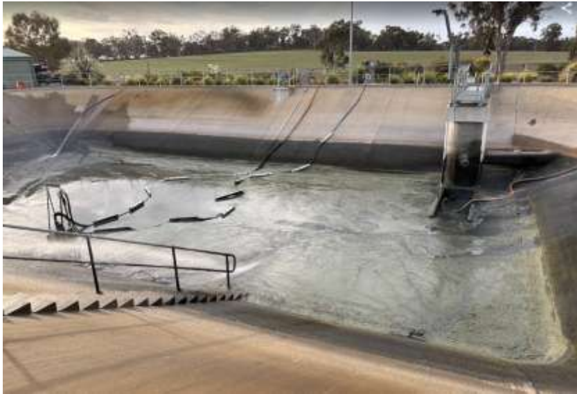
Sludge in the balance tank at the Mulwala WMF prior to cleaning
