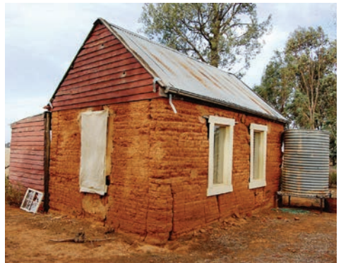
Pictured above: Before restoration, the hut was threatened by severe structural cracking.
